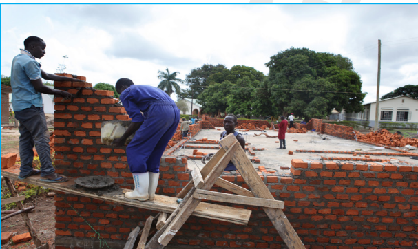
Construction of the physiotherapy unit.
