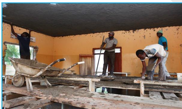
Renovation of the children's village.
