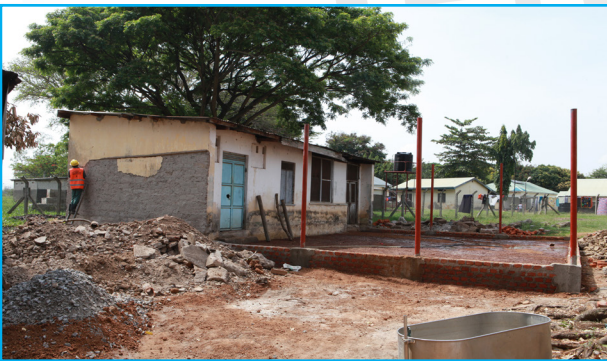
Construction of the orthopaedic fabrication workshop.
