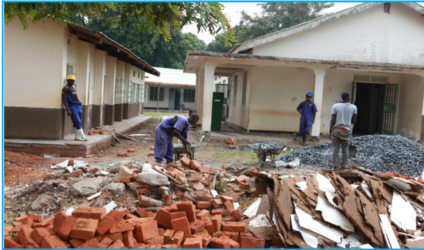
Construction of the eyeward OPD
