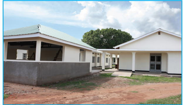
Renovation of the eyewards
