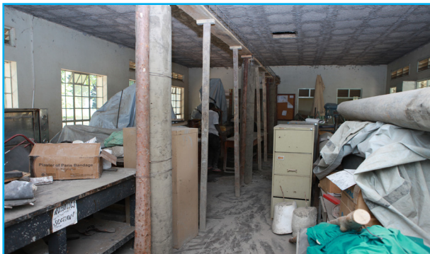
Renovation of the orthopaedic workshop.
